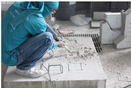
Fig. 8. Removing concrete via drilling machine.
