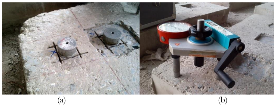
Fig. 10. Installing pull-off test: (a) the steel disk; (b) the tensile loading device.
