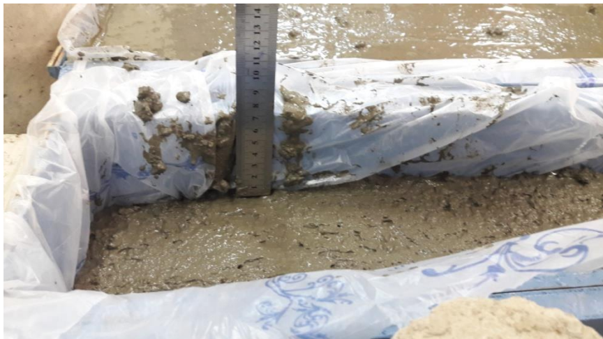
Fig. 3. Layered casting of concrete beam specimens for steel fibre alignment.
