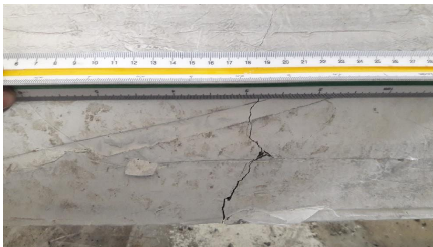
Fig. 14. Thin crack width in double hooked steel fibre concrete (DHA-10).
