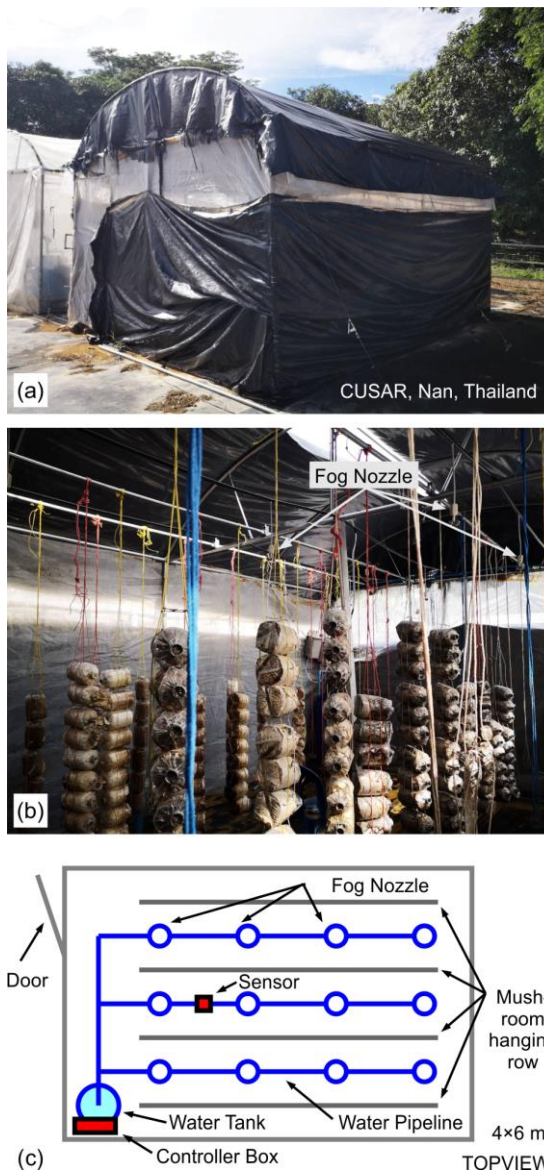
Fig. 1. Photos of the developed mushroom cultivation house (a) outside and (b) inside. In (b) three fog nozzles are pointed by arrows. (c) Top-view schematic of the installed fog nozzles, mushroom hanging row, 200-liter water tank, water pipelines, temperature/humidity sensor and controller box.
