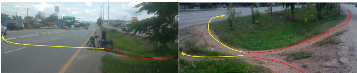
Fig. 6. An illegal movement at the drainage ditches on the median of the road.
