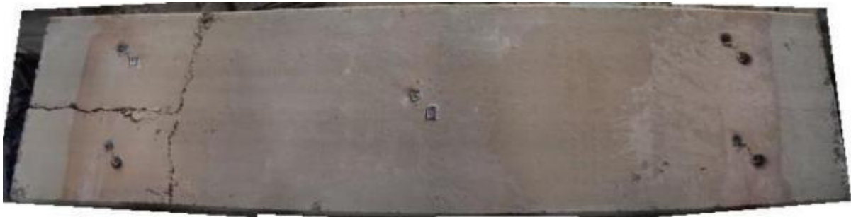
Fig. 17. HCL4 after fire test.
