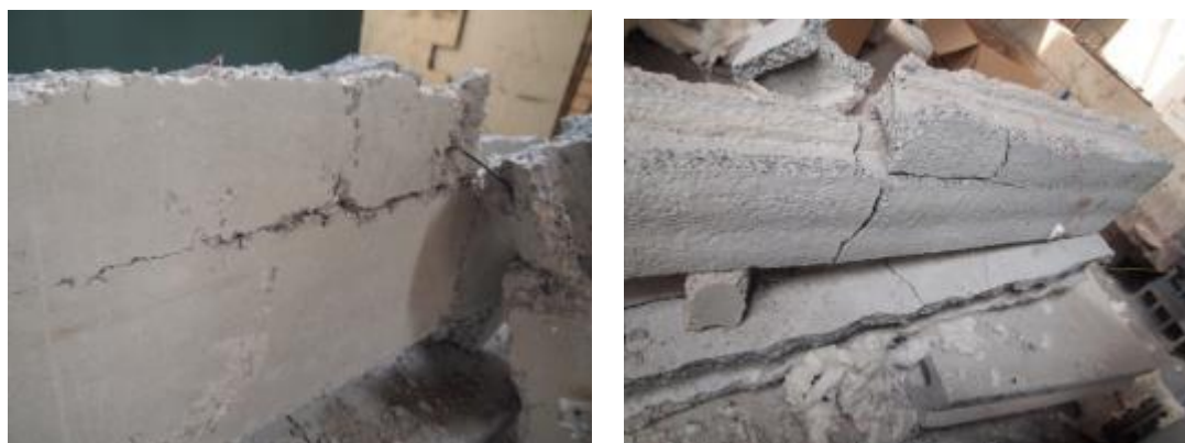
Fig. 19. HCL6 after fire test.
