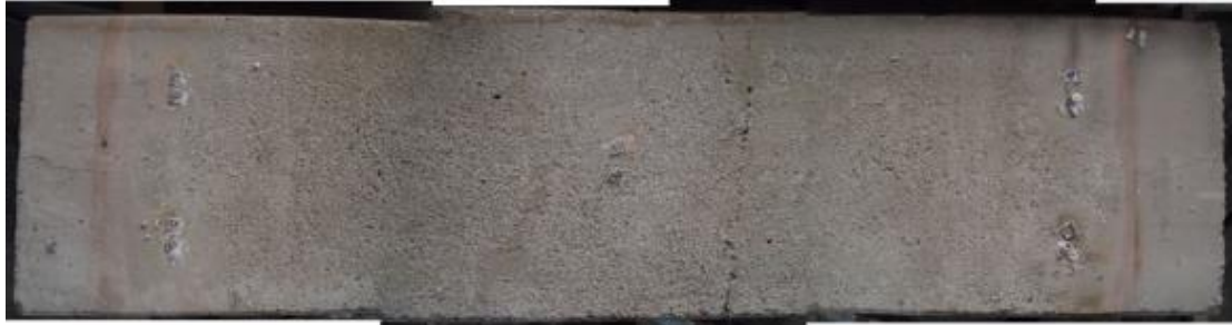
Fig. 15. HCL2 after fire test.
