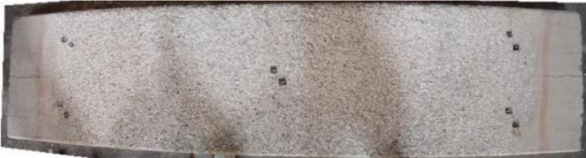
Fig. 16. HCL3 after fire test.
